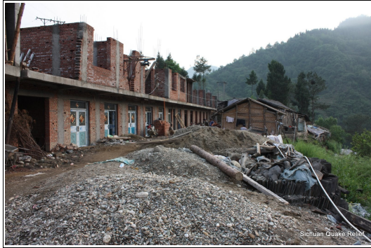
New housing stands unfinished, in front of temporary accommodation. (May 2010)
